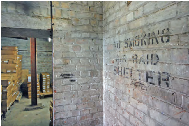
In the reused cellar of a Manchester city centre shop, some simple shelter rules greet arrivals at the base of its wartime external stairs. Steel structural reinforcement, added to withstand the load of the collapsing building above, survives beyond
